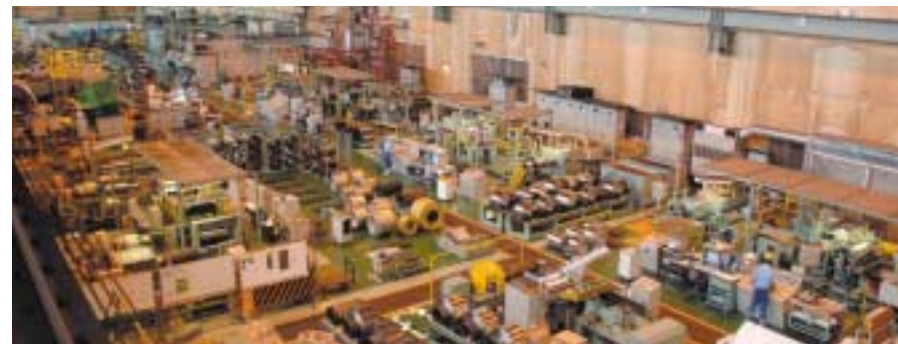
Full view of stainless foil plant (Ichikawa Works)
