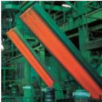
Kure Works' continuous casting facilities
